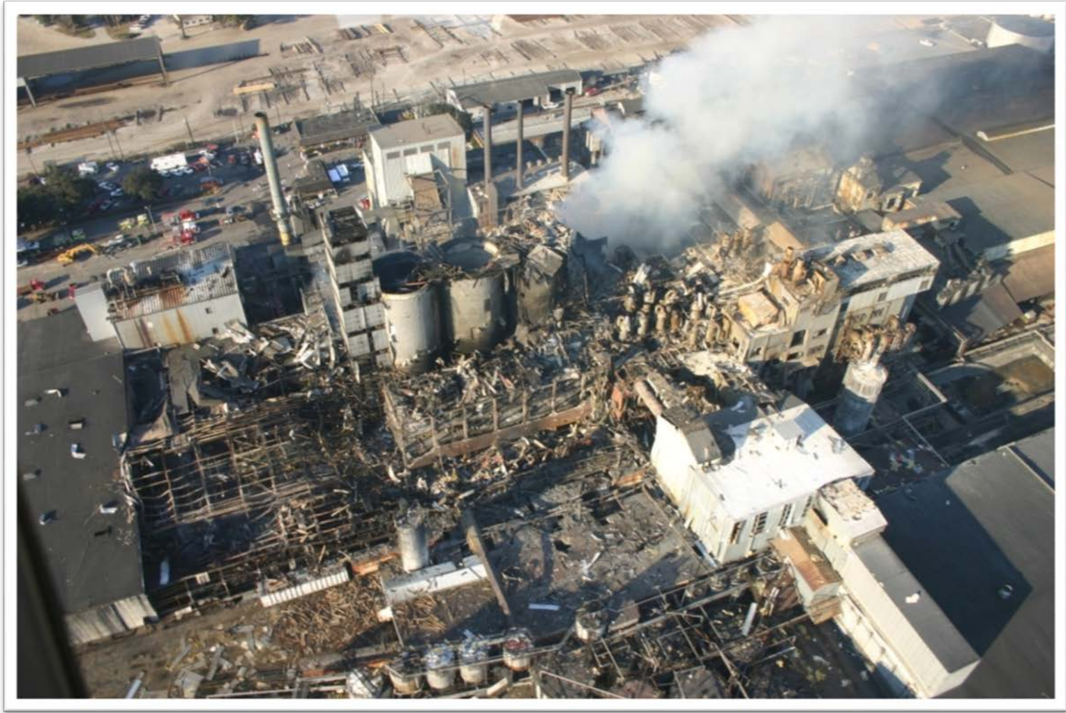
Photo: U.S. Chemical Safety Board
